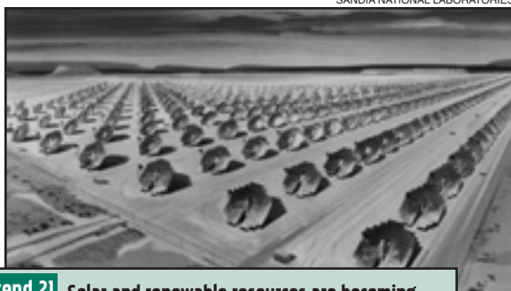
Trend 21 Solar and renewable resources are becoming more competitive with oil. Pictured is a solar dish-engine system (artist's concept) under development by Sandia National Laboratories and Stirling Energy Systems Inc.
